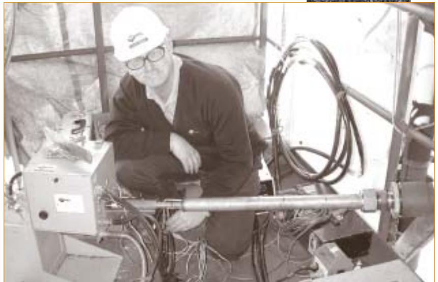
Environmental consultants, HRL Technology, sample flue gases for analysis. The continuous sampling takes place prior to the final gas cleaning unit
