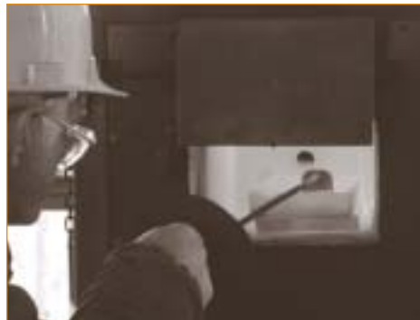
Ernie Walpole conducts calcining tests on SR product
