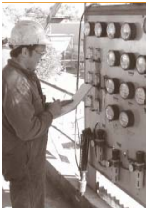
John Winter logs pressure readings to verify fluid bed roaster performance
