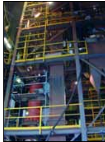
LTR roaster construction in New Zealand
