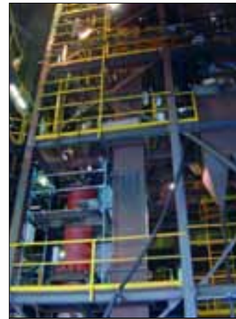
LTR roaster construction in New Zealand
