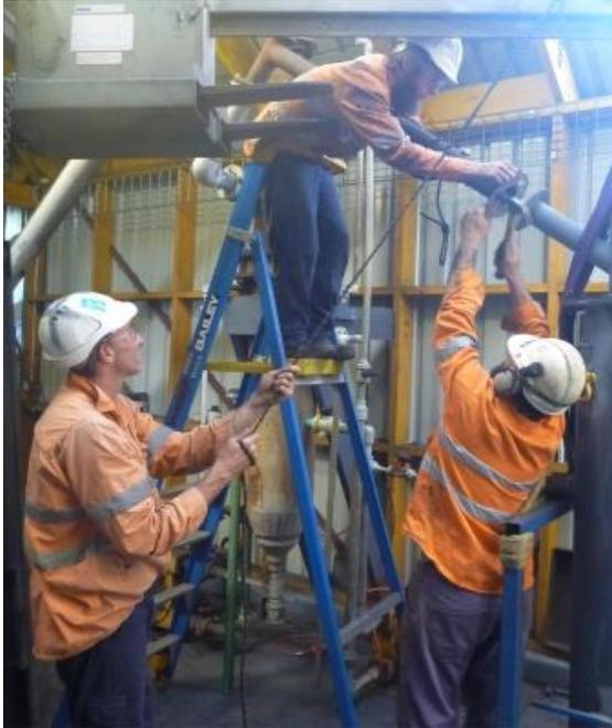
**Installing the gas duct from the batch fluid bed roaster to the venturi-scrubber**
