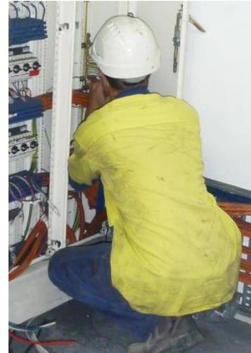
**Connecting the electrical controls for the air compressor**
