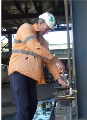
**Installing outlet valves on the HP air lines in the North Tower**
