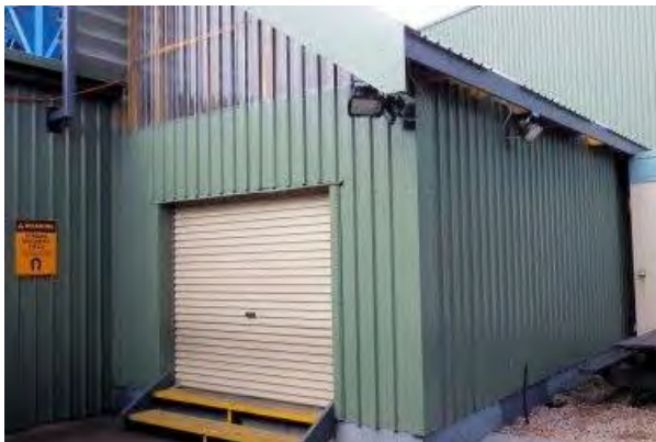
Construction of the new laboratory is complete and at the lock-up stage.
