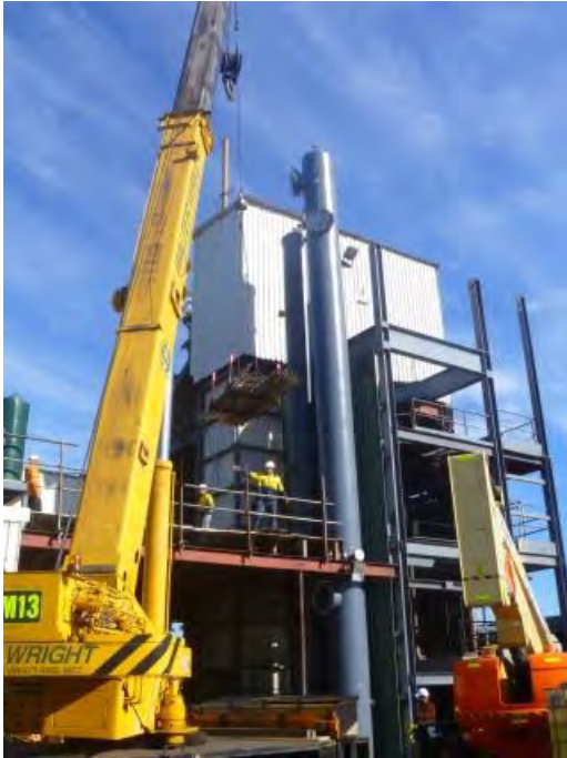
Installing the CO 2 stripping and absorption columns.
