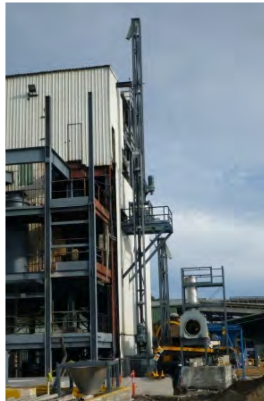
The Olds elevators to transfer mill scale from the pre-treatment area into the Plant are installed.
