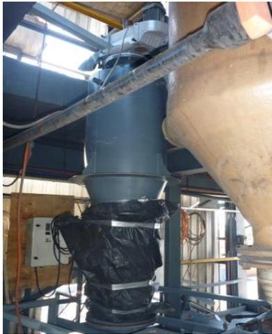
**Fluid bed evaporator to produce mixed iron oxide/chloride pellets for pyrohydrolysis (acid regeneration)**
