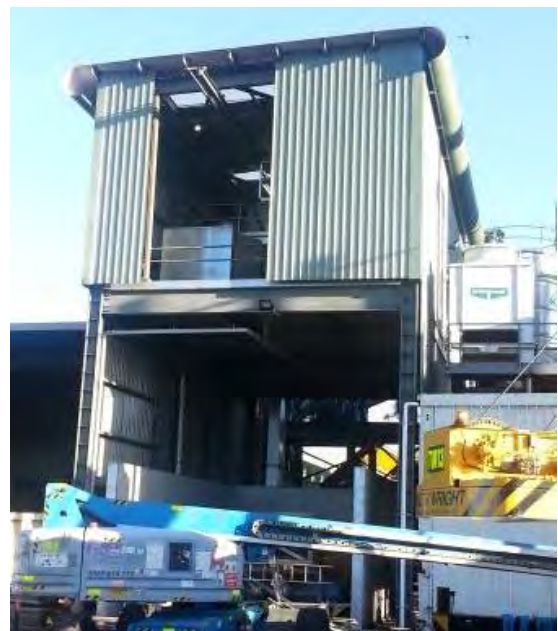
The completed plant room above the iron briquette product load-out bunker
