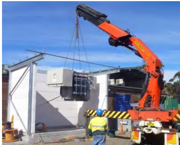
Installing the high voltage transformer
