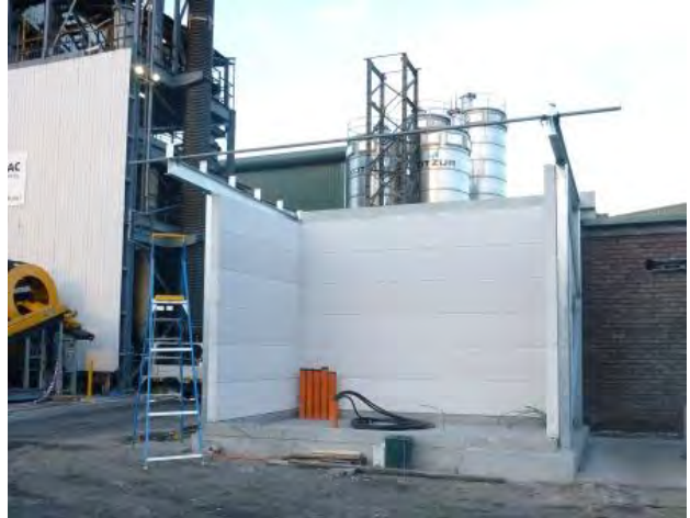
Construction of the fire-proof building to house the 33 kVA transformer
