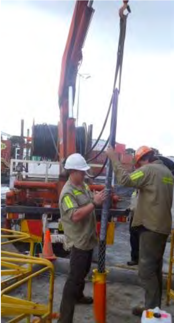
Drawing the 33 kVA cables from the HV transformer to the HV switch room
