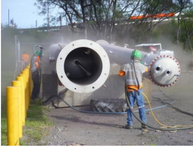
CO 2 stripping columns being sandblasted and coated prior to installation
