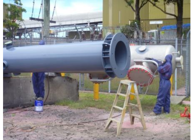
CO 2 stripping columns being sandblasted and coated prior to installation
