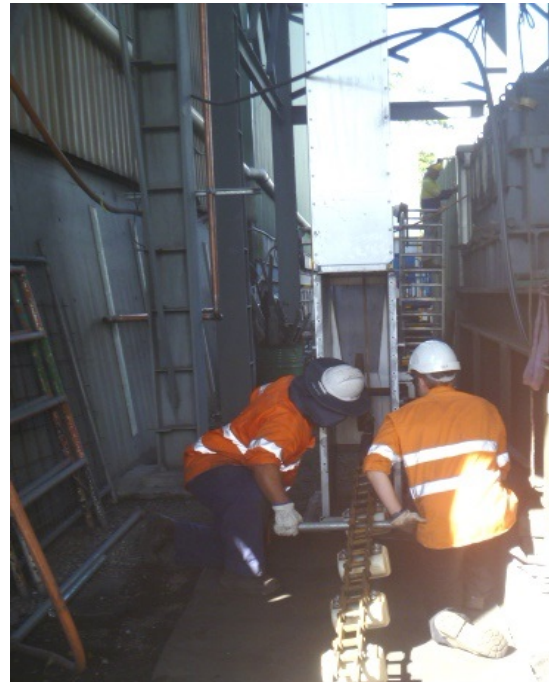
Installing the bucket elevator chain
