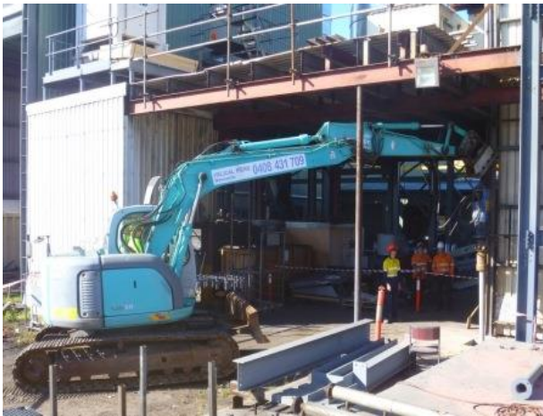
Installing screw piles to support the CO 2 stripping columns
