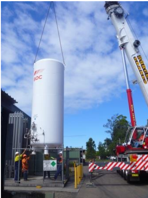
Installing a larger nitrogen storage tank
