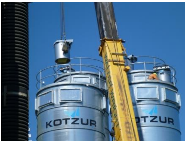
Installing the dust filter
