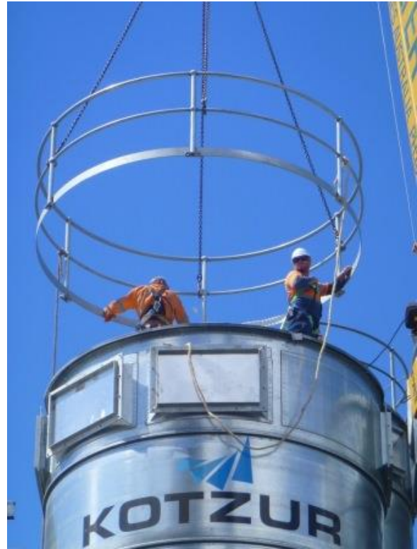
Installing safety handrails
