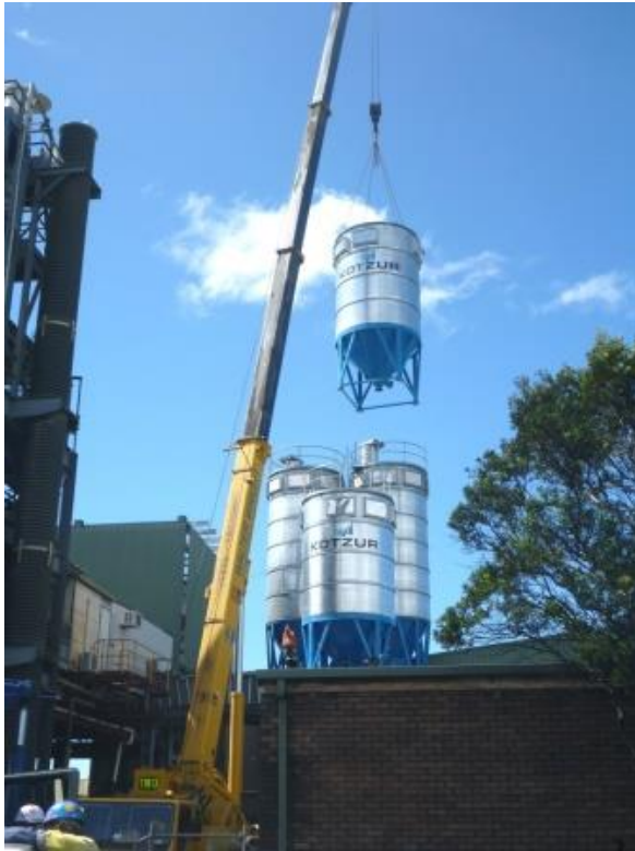
Installing the silo for the reduced iron product
