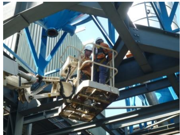
Final check of silo installation
