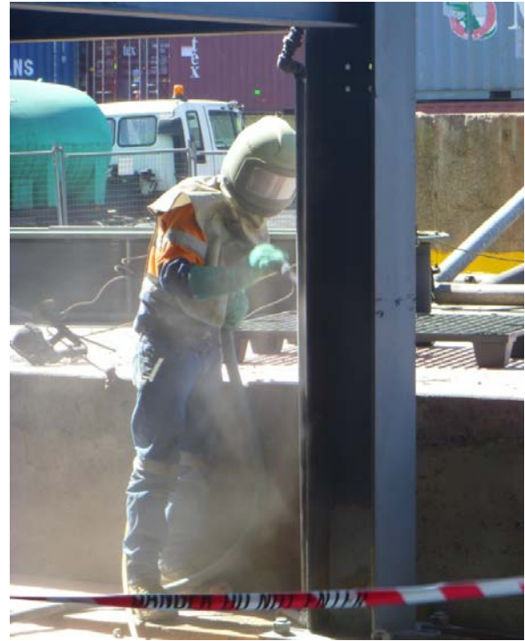
Preparing steel columns for epoxy coating
