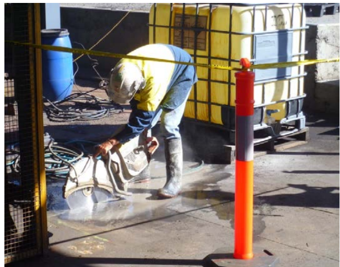
Preparing foundations to support the CO 2 stripping columns
