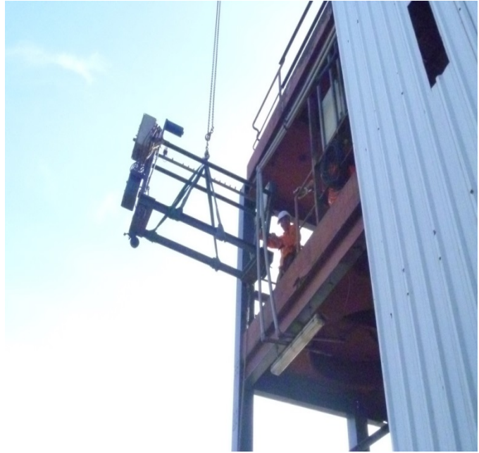
Installation of the frame for the plate filter
