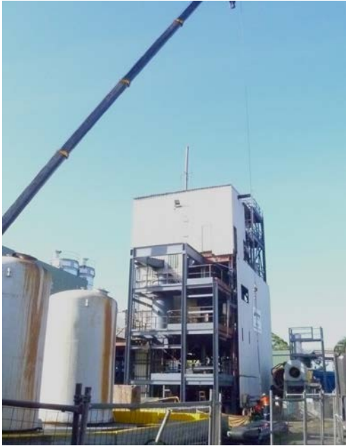
Preparing to lift equipment into the process tower
