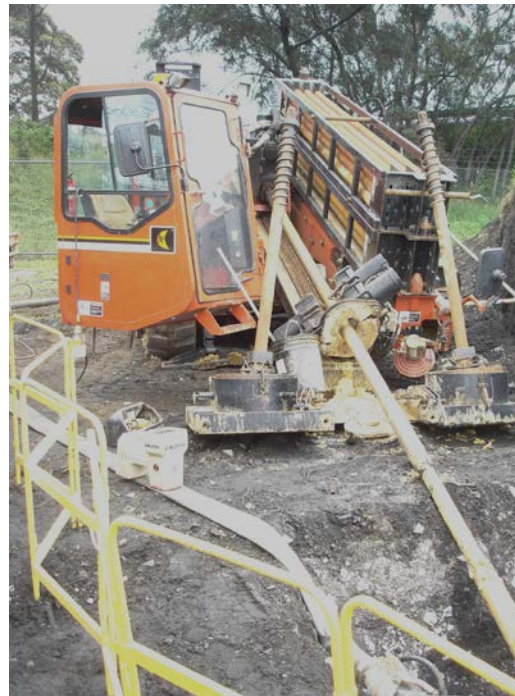
Horizontal boring machine installing conduit for high voltage cable
