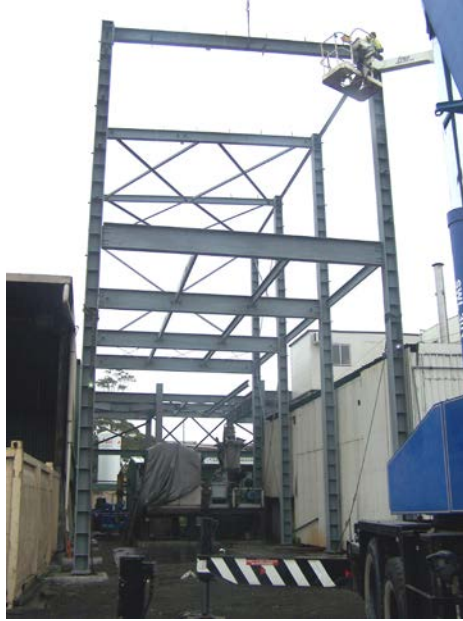
Left: Construction of structure for Koeppern briquetter (at rear), iron briquettes load-out bin, and elevated plant room
