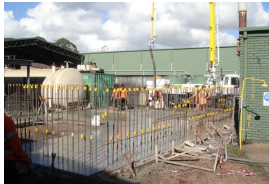
Floor of bulk mill scale storage shed
