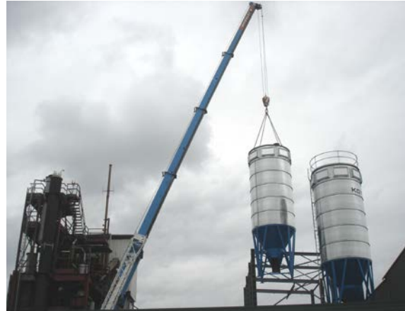
Installation of binder silos
