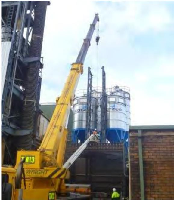
**Installing the lower section of the tower to support the magnetic separator (to separate iron chips from char before the products are diverted to their respective silos)**
