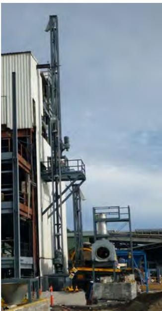
Mill scale is fed to the Plant via the Olds elevators installed on the western wall
