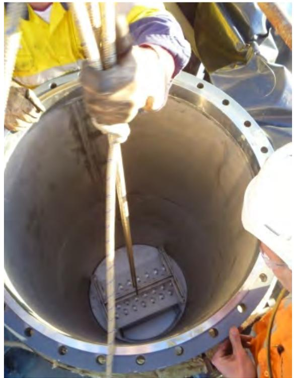
**Installing the trays into the columns**
