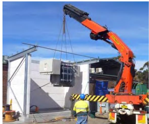
**Installing the 33 kVA transformer in the fire-proof building prior to roofing**
