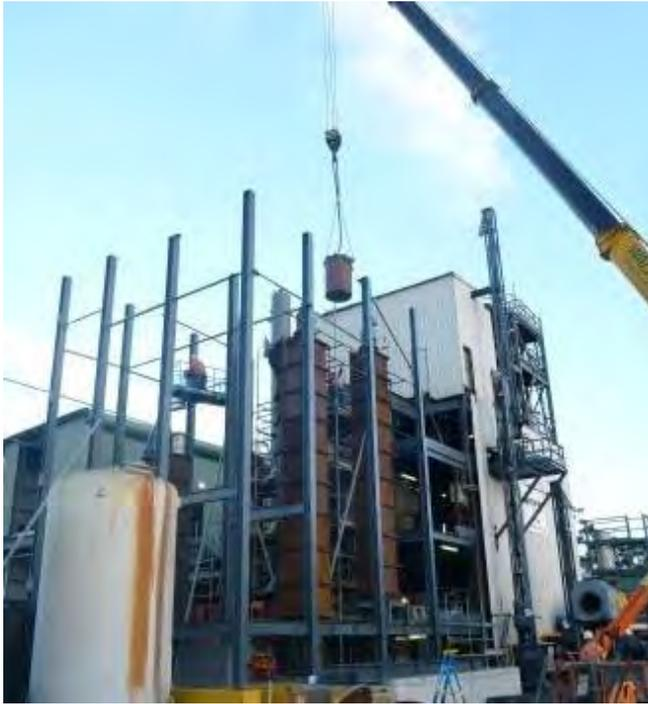
**Hoisting the fibreglass tank which will hold strong acid into the north tower**
