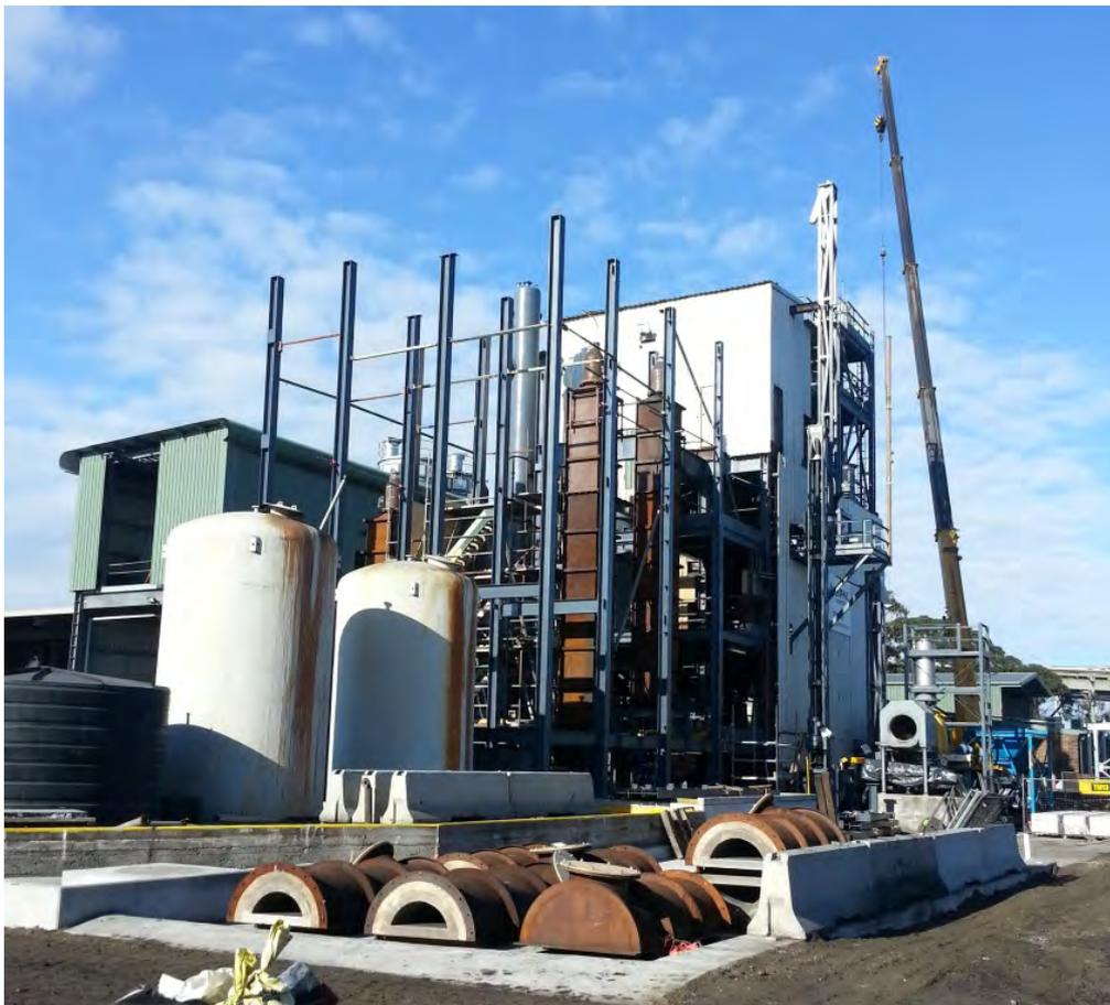
**View of the Plant from the northwest, showing the mill scale handling section on the western wall, the structural steel for the north tower extension with the stove shells in position, the stove front covers stored in the completed bunded tanker delivery area (foreground), and the completed Plant services room (upper left centre)**
