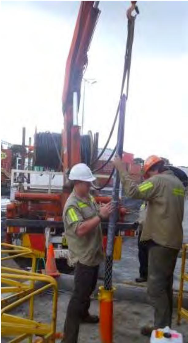
**Drawing the cables from the HV transformer to the HV switch room for the 33 kVA power supply**
