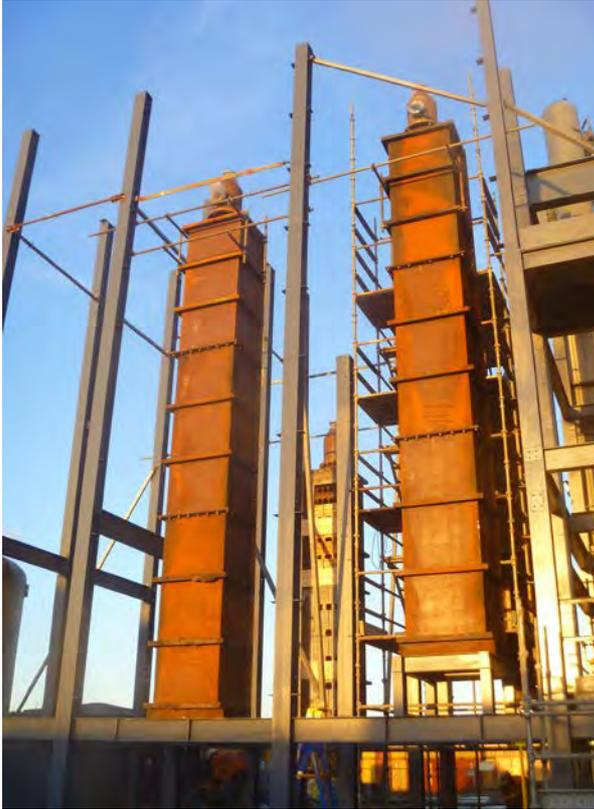
Installation of the four stoves for heat recovery and transfer in the north tower is complete
