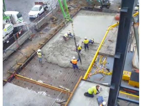
**Pouring the slab for the bunded pickle liquor delivery and regenerated acid load-out area**
