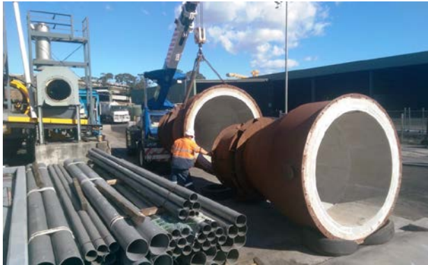
Positioning the roaster bodies alongside the Plant
