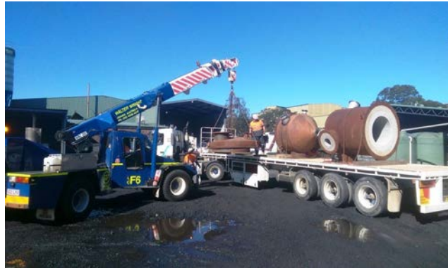
Unloading the roaster caps and plenums (bases)
