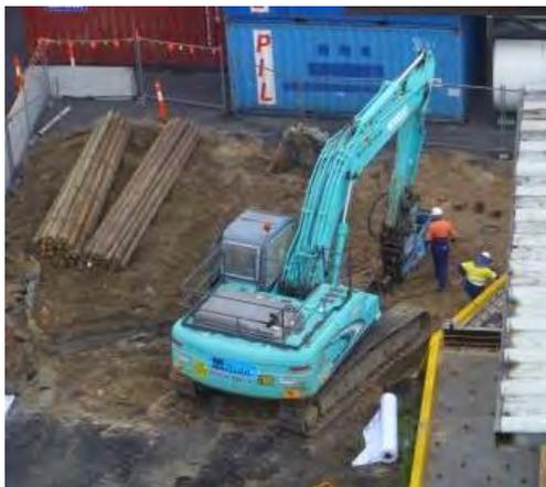
**Excavation is underway for the tanker loading area sump tank, adjacent to the tank farm**
