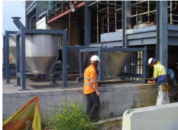
**The Olds elevators (left) and associated hoppers (right) have been delivered. These will be used to transfer both mill scale and coal held in bulk storage into the Plant and will be installed in the coming quarter**
