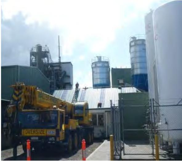
The bulk nitrogen and oxygen supply (right side of the photo) has been reticulated to the Plant, and the laboratory roof and the silos have been installed. The existing ilmenite leaching section of the plant is to the left rear of the photo
