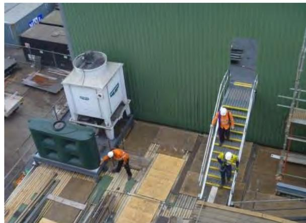
**The cooling tower and feed water tank have been installed, as well as the permanent access stairs to the plant room**
