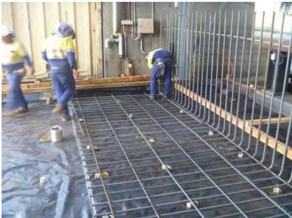
Installing reinforcing for floor and walls of the iron briquette product load-out bunker
