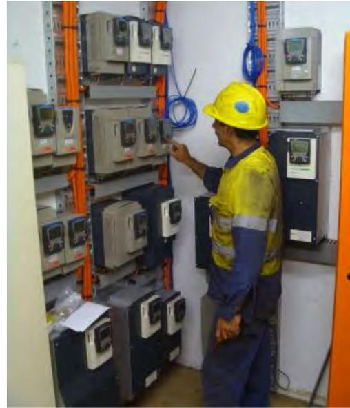
**The motor control room houses the variable speed drives which control the fans and blowers that supply air to the Plant**
