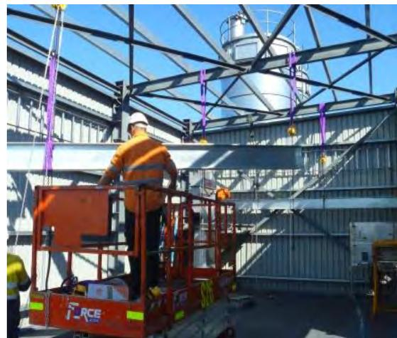
**Installation of the mezzanine floor in the plant room is underway. This will support air blowers and compressors**
