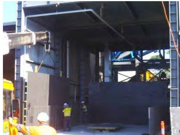
Installing formwork shutters for the walls of the iron briquette bunker after the concrete floor has been poured
