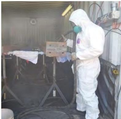
**Sandblasting operations underway in the modified shipping container**
