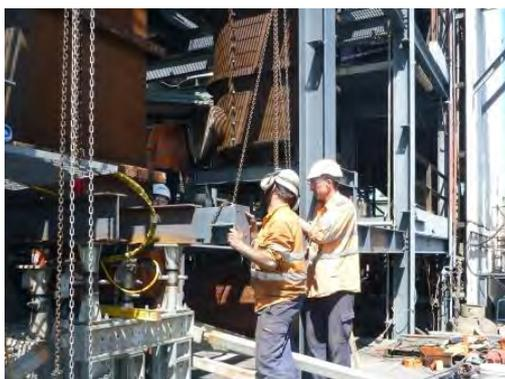
**Installing the cross member beams in Level 6 of the North Tower**
