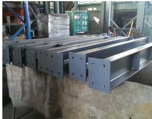
**Painted beams prior to installation in Level 6 of the North Tower**
