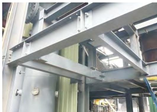
**Completed installation of Level 6 support beams**
