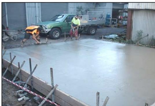
Reinforced concrete slab foundation for briquetter.
