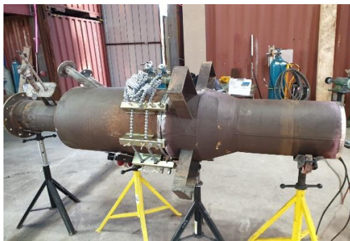
Fluid bed roaster repairs are underway at Compass Engineering's workshop
